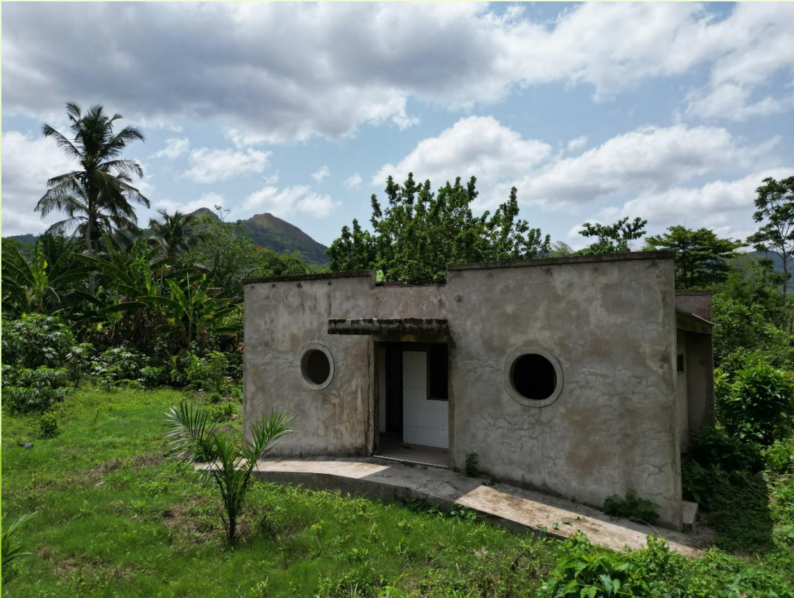
Toilet Facility - Liati Tourist Pavilion
