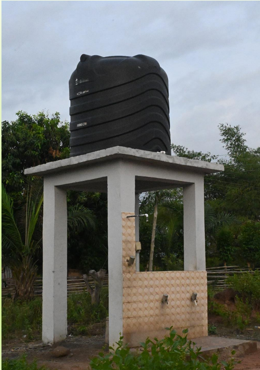
Mechanised borehole - Ve Golokuati
