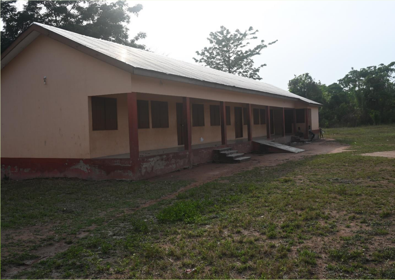
3 Unit Class room block | Ve Koleanu
